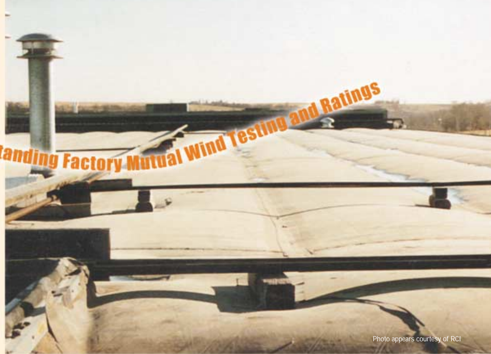
Membrane billowing between points or lines of attachment.
