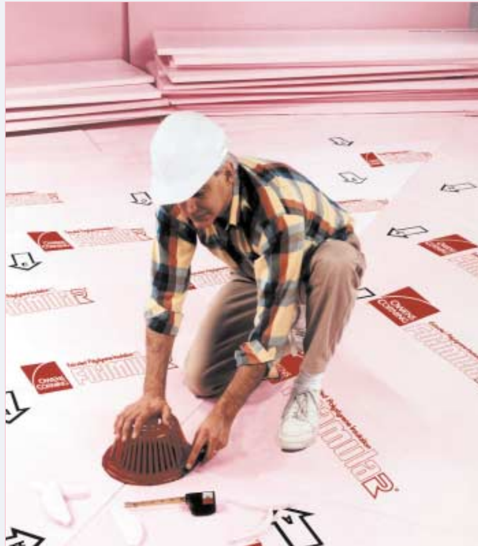
When a tapered insulation system is provided, insulation boards are marked with letters and directional arrows that tie into layouts provided by the manufacturer.
